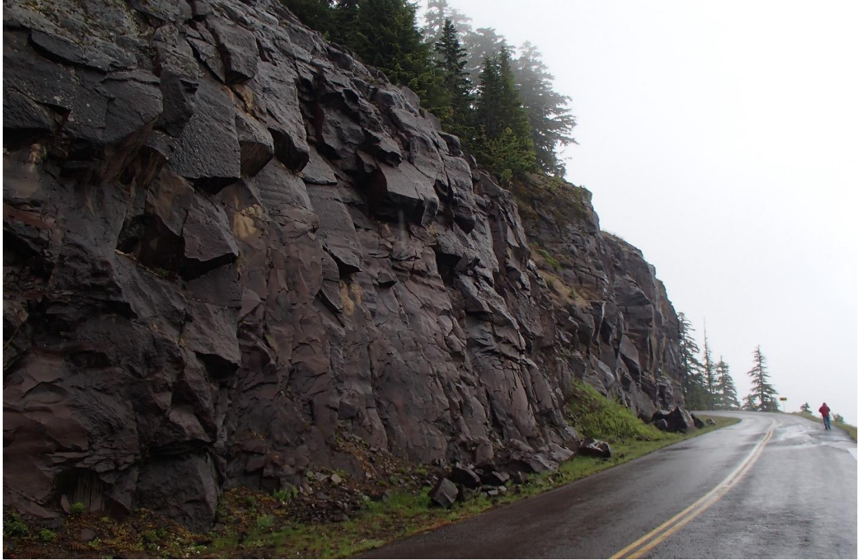
Figure 2-6: Rockfall debris in the roadside ditch can be used to help assess both block size/event volume and failure type. Forest Service Rd 25, Milepost 25.
