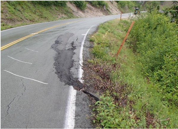
Figure 2-3: Roadway deformation caused by embankment failure. Forest Service Road 90, Milepost 11.5.
