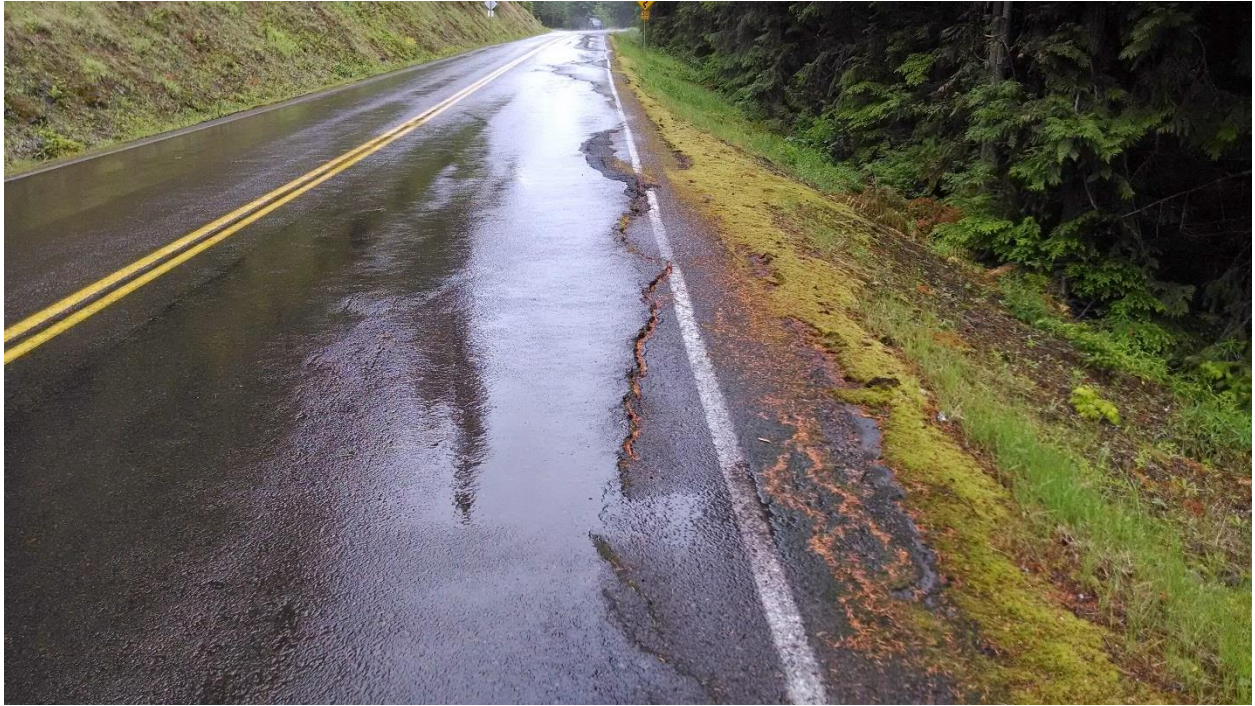
Figure 2-1: Embankment failure affecting up to 25 percent of the roadway. Forest Service Road 25, Milepost 30.
