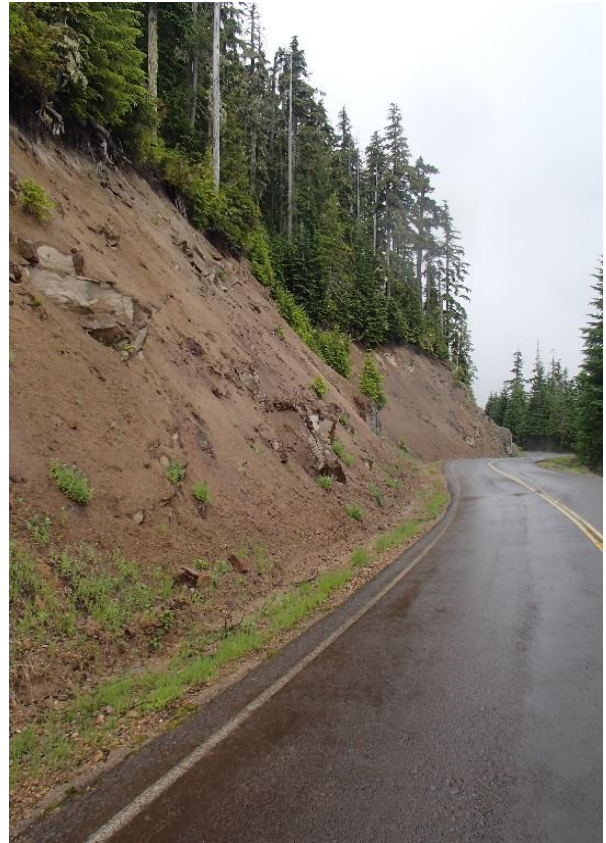
Figure 3-7: Rock cut where differential erosion is the dominant cause of failure. Forest Service Road 25, Milepost 30.
