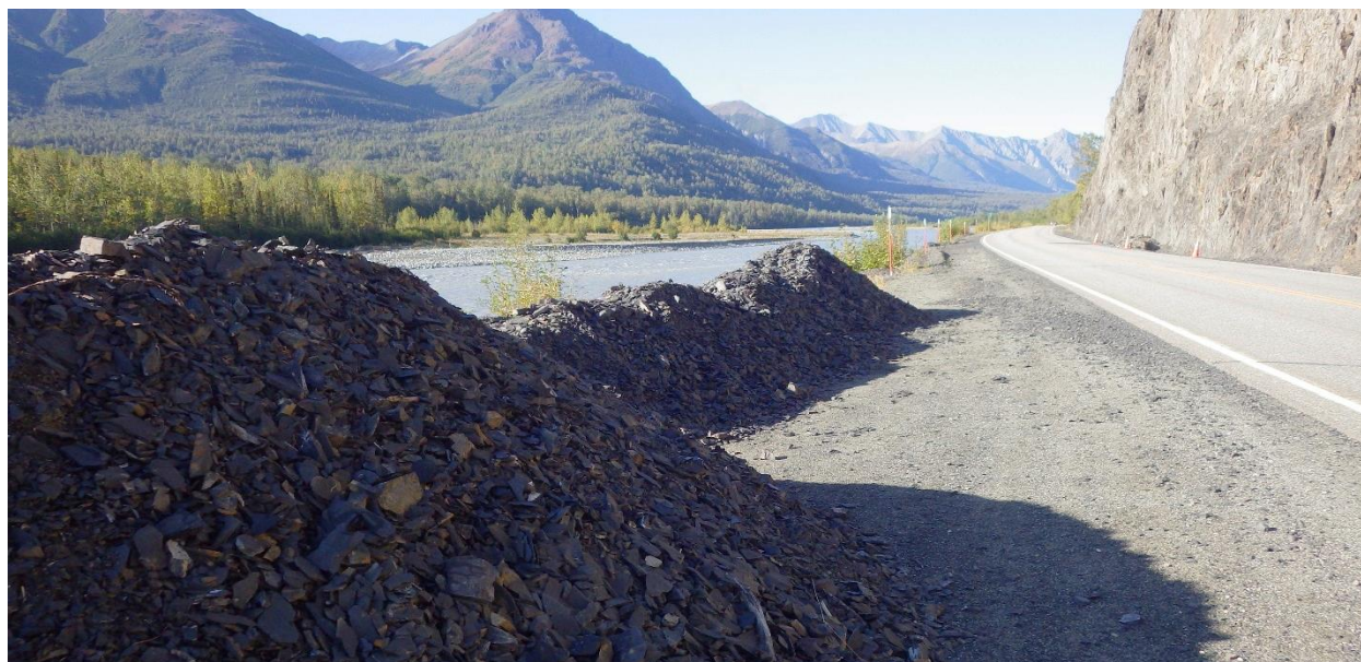
Figure 3-5: Constant rockfalls occur at this rock slope on the Glenn Highway in Alaska. Maintenance personnel stockpile the daily debris in this pullout for regular removal. This rock cut received a category score of 100.
