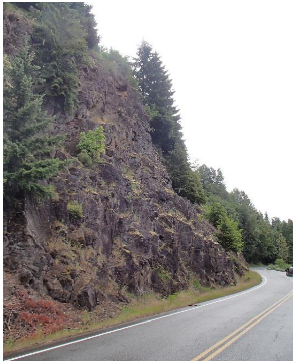
Figure 3-6: Rock cut where failure is controlled by interaction between geologic structure and rock friction. Forest Service Road 90, Milepost 13.
