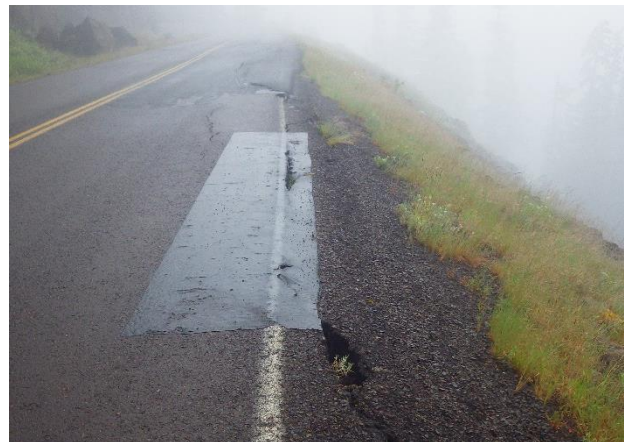
Figure 3-4: Instability requiring repeated maintenance attention. Forest Service Road 25, Milepost 25.
