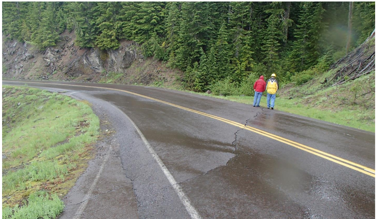
Figure 2-2: Embankment failure affecting entire roadway. Forest Service Road 25, Milepost 25.
